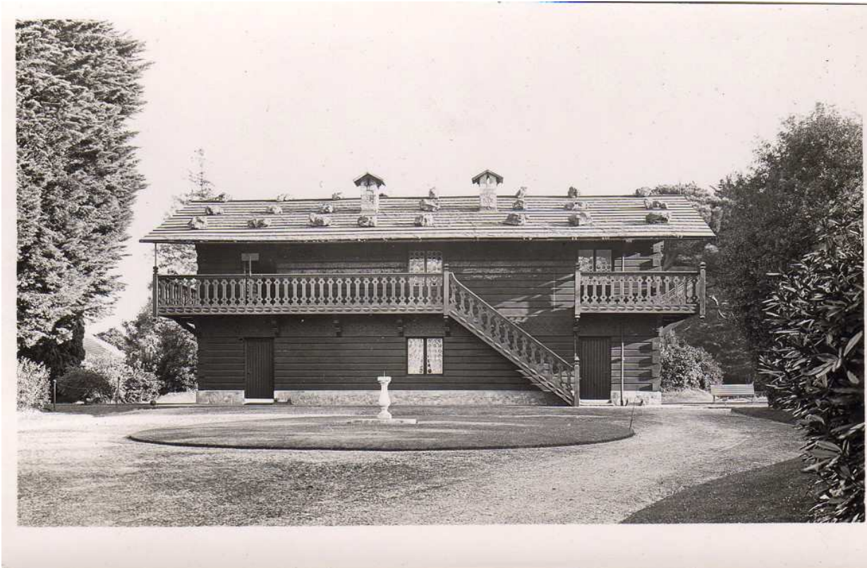
Photograph of the Swiss Cottage, north elevation, pre 1934.
